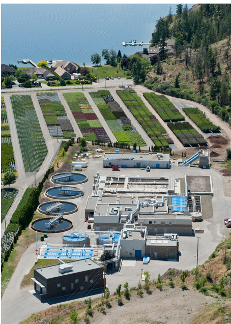
Westside Regional Wastewater Treatment Plant located off Gellatly Road in West Kelowna. Photo courtesy of RDCO.
